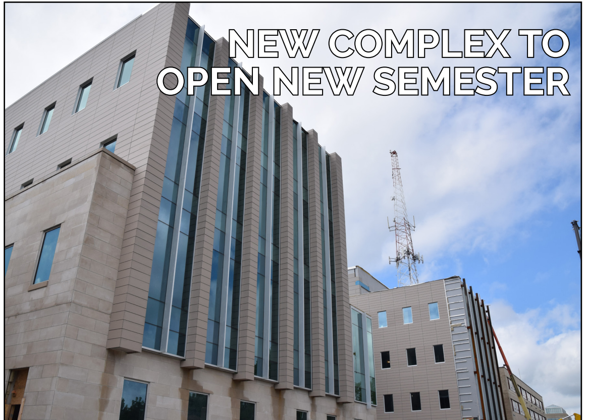
Costing over $100 million, the Business and Engineering Complex project broke ground the summer of 2017. Current phase one of the complex is set to open in August for classes. photo by Tony Xu
